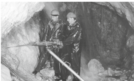
Construction of Schneealpe gallery
