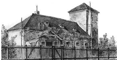
Duke Albert Water Pipeline
