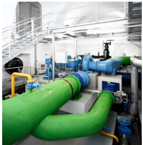
Part of the water transported to Vienna via the 2 nd Spring Water Main is used for electricity generation by driving a Francis turbine situated in the Mauer power station.
